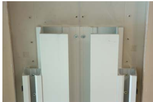
Figure 4.1b. Staggered Track and Chain Guide Joints
