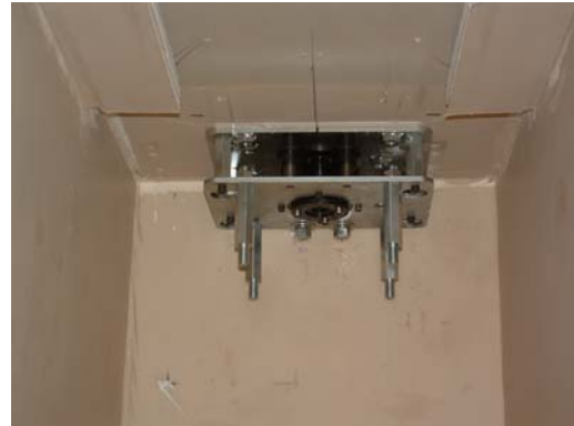
Figure 1a. Centering Operator Mount
