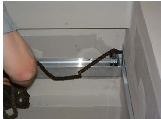
Figure 3.5a. “Threading” End Sprocket Assembly
