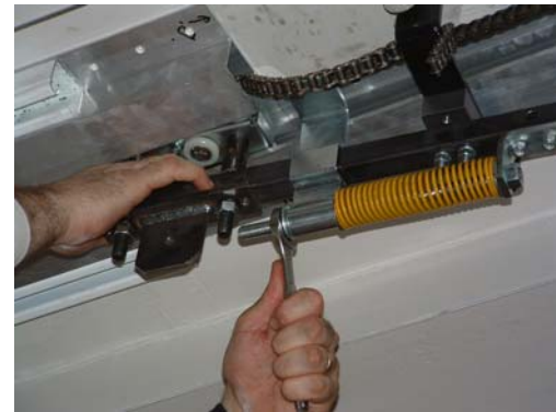
Figure 3.6. Adjusting Chain Tension
