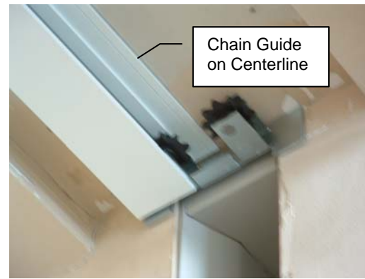
Figure 3.1. Chain Guide Loading Section and Sprocket Assembly
