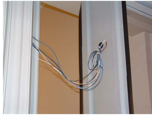
Figure 12b. Leaving Extra Wiring
