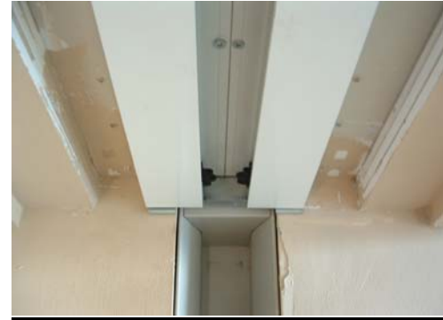
Figure 3.2. Installed Loading Section
