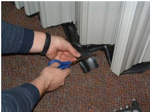
Figure 14a. Trimming Sweep from Outside
