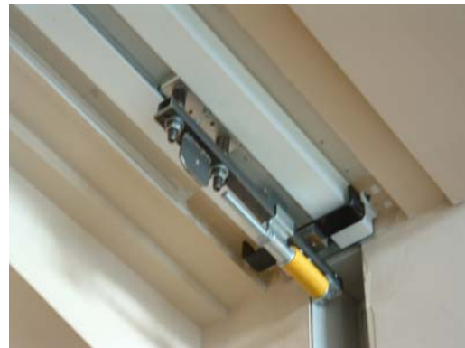
Figure 6.1. Trolley in Position for Loading Curtain
