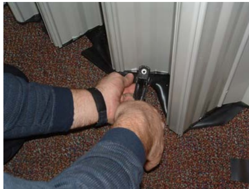
Figure 14b. Joining Sweep from Outside
