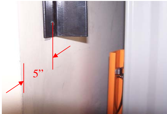
Figure 15. Jamb Stop and Exit Hardware
