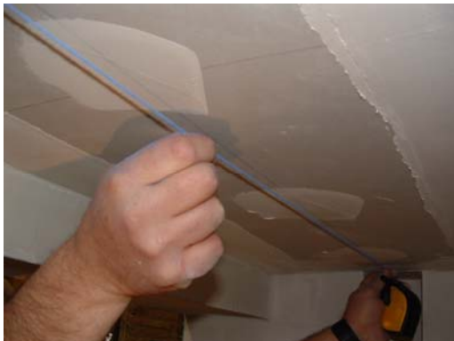
Figure III.1. Marking the Centerline
