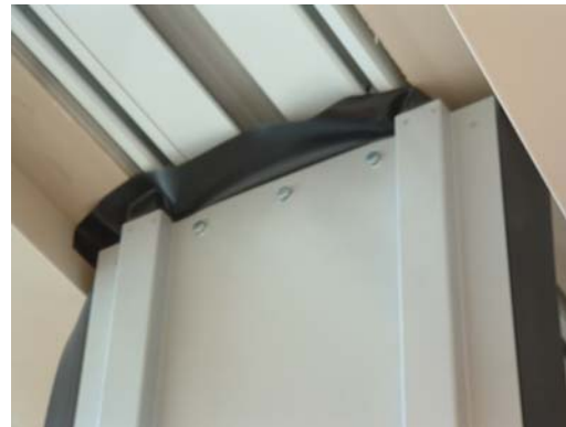
Figure 7b. Installed Floating Jamb & Fasteners
