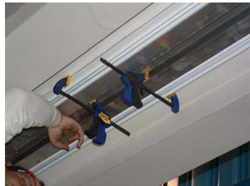
Figure 3.5b. Using Clamps to Secure Chain
