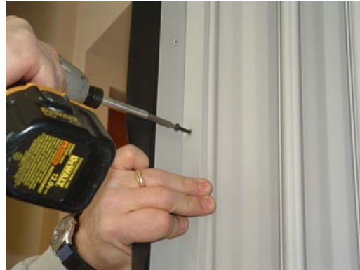
Figure 11. Attaching Jamb Section to Floating Jamb
